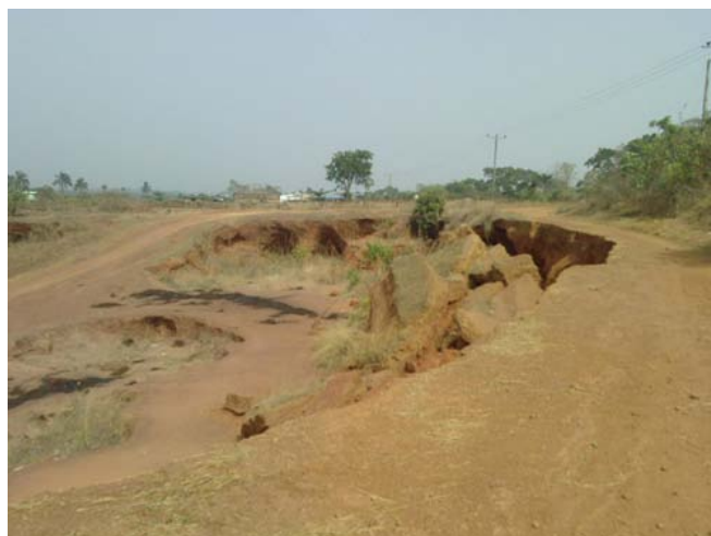
Plate 1: Erosion site in Anyigba, Nigeria
