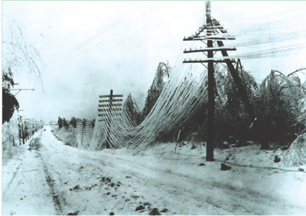
Figure 2 Wires with Accrued Ice
